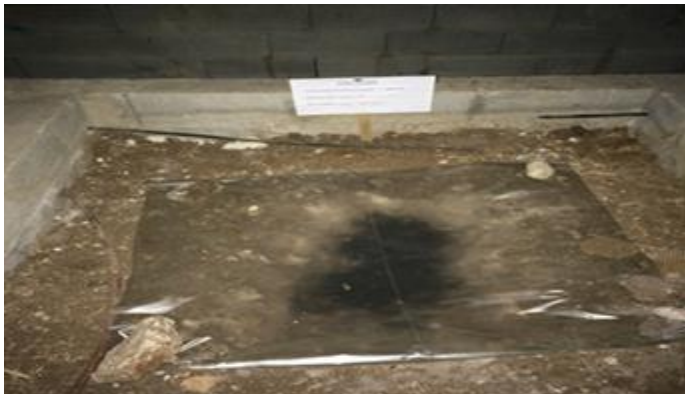
Figure 3-1: One of Piles used in 1st stage
